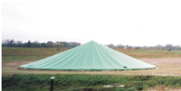
Figure 2. Urine reservoir with a light roof on A. Visockas farm in Biržai district.
